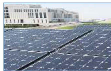
GU Tech – Eco House (Oman) 12Kwp Grid Connected System
